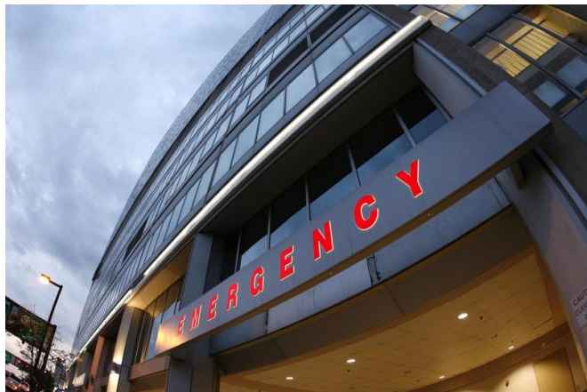
Hahnemann University Hospital Emergency Room at dusk. Credit: Hahnemann University Hospital
